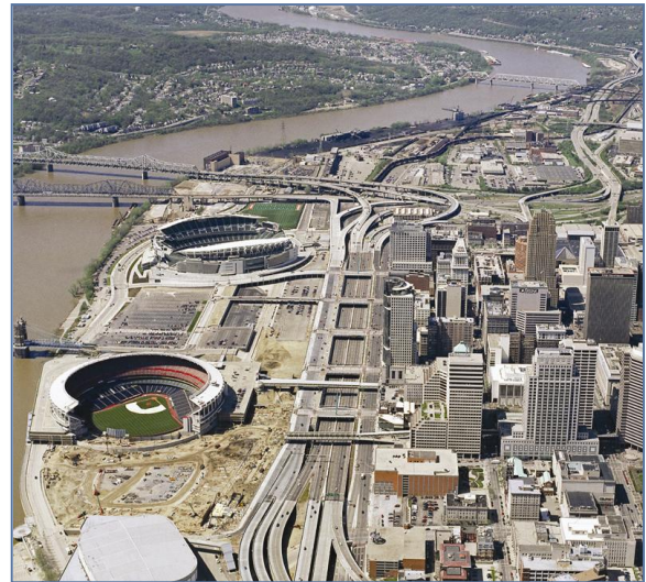
This project involved a comprehensive reconfiguration of a depressed highway – I-71 (Fort Washington Way) in downtown Cincinnati.
