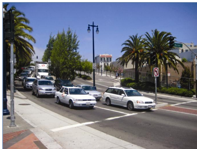
In this project, San Francisco’s Central Freeway was replaced with an urban boulevard (Octavia Boulevard).
